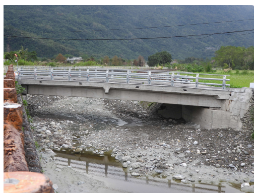
114.01.16/欲改善之橋梁現況
